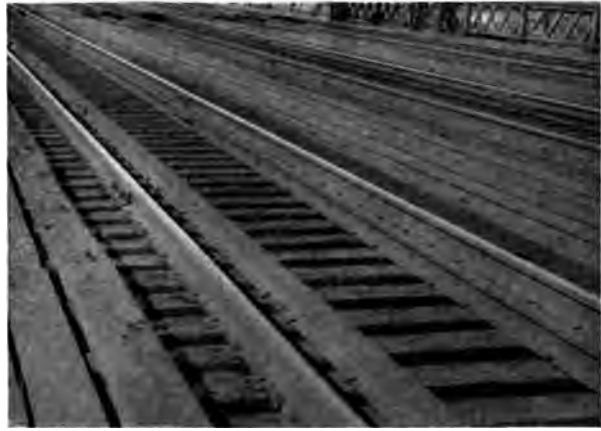
P. & M. Rail Anti-Creepers on the Erie Railroad on Viaduct Approaching Bergen Archways, Jersey City, N. J.
